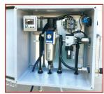
Control panel will allow operator to increase air flow and change speed of pulsating
